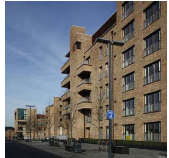
Modern use of brick in an historic environment—McEwan Square / Fountainbridge Brick has been used to integrate this development into its historic surroundings. The development is overtly contemporary in its appearance. The colour of bricks was chosen to harmonise with the stone of the adjacent tenements. Combined with the vertical emphasis to the window and the building's scale, the material choice has helped ensure this development adds to Edinburgh's sense of place. This development sets the standard for the use of brick within Edinburgh.
