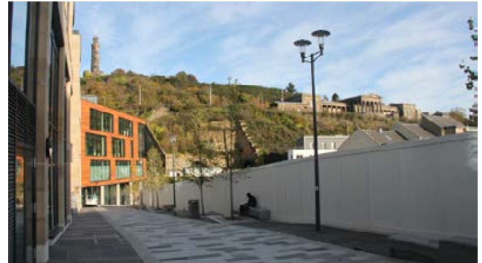
New public realm and link created between Canongate and Calton Road (the building on the right is still under construction).
