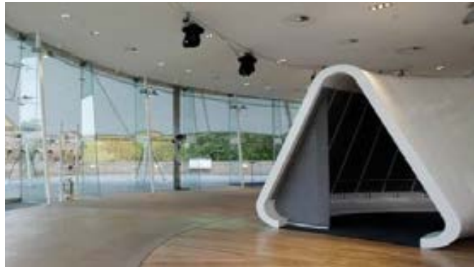
Good design for noise was used at Our Dynamic Earth to stop noise escaping from one of their function areas. Instead of installing doors they installed a triangle, zigzagged corridor.
