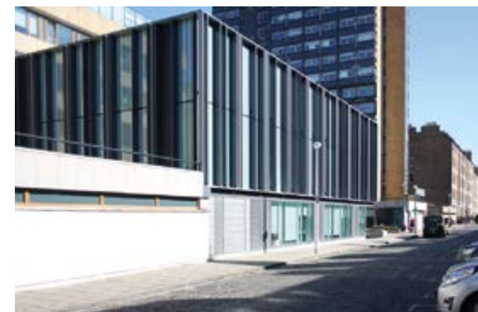
Curtain Walling - Buccleuch Place The potential offered by glazing systems with variations in the window widths, patterning of the glass and mullion depths is fully taken advantage of here.
