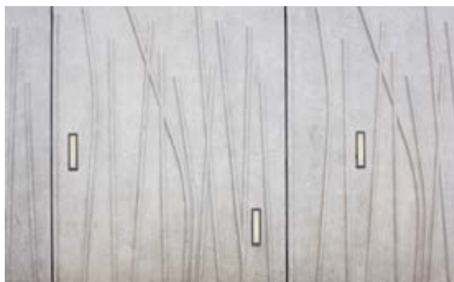
Concrete used sculpturally—Horse Wynd The sculptural potential of concrete is exploited in the Parliament wall with the patterned surface and integration of lights
