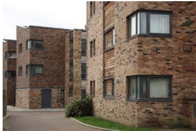
Subtle variation—Telford March Two different mixes of brick have been used to provide variation in colour within the elevations.
