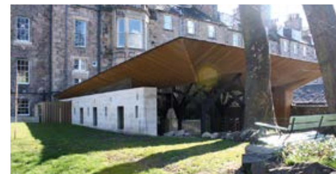
Frameless glazing - George Square Lane Glazing is used to create the effect of a floating roof on this building.
