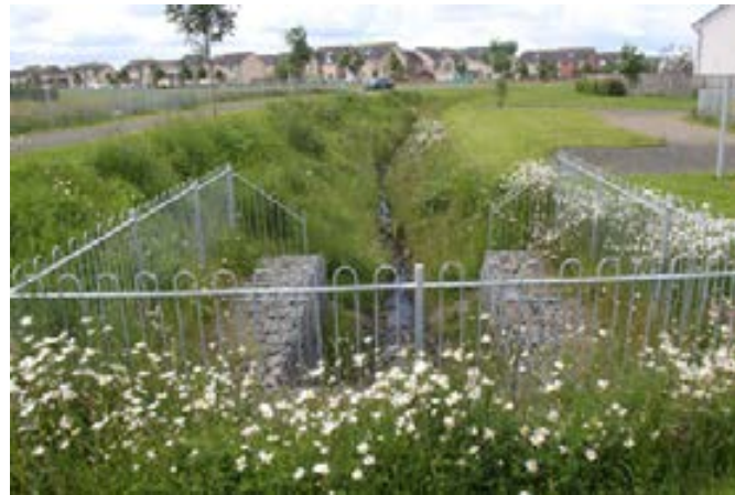
SuDS retention basin and swales, Kirkliston
