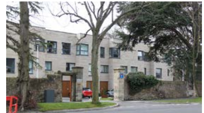
Boundary walls in villa areas—Newbattle Terrace Boundary walls are extremely important to the character and appearance of villa areas. The size and number of new openings to them should be minimised.
